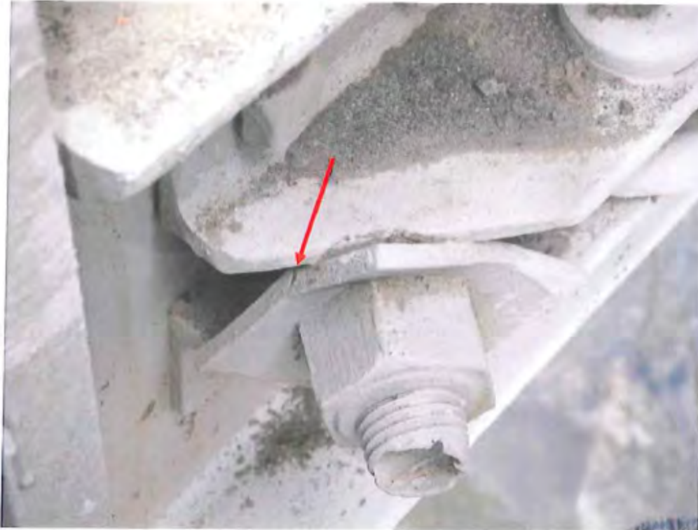
PHOTO 27 - CRACK IN LATERAL BRACING CONNECTION WASHER AT L4, UPSTREAM
