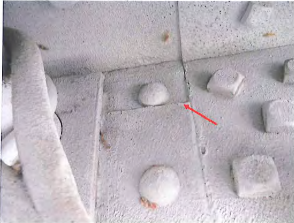
PHOTO 12 - CRACK IN UPPER CHORD OUTER WEB NEAR U5, DOWNSTREAM
