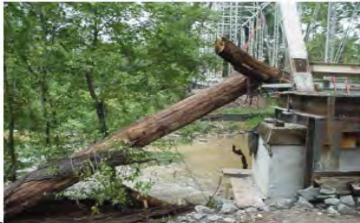
Tree Impact on Metalized Truss (Reconstruction in 2003)
